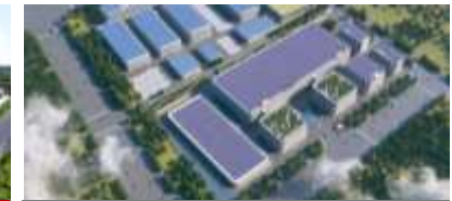
Plant 4 Luohe Factory #2 (Under Construction)
